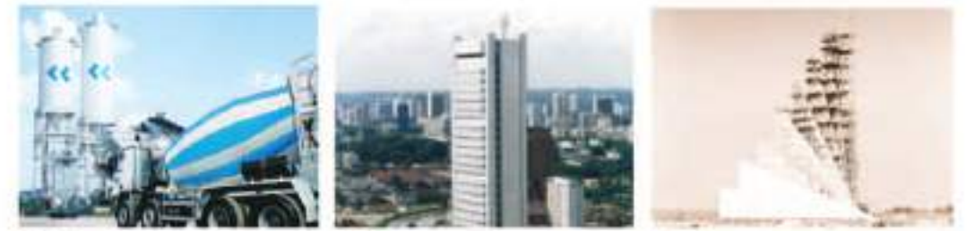
1990 First Concrete Batching Plant of Bangladesh was set up by Concord 1984 Constructed Telecom Building in Singapore 1982 Constructed National Martyrs' Monument in only 89 days
