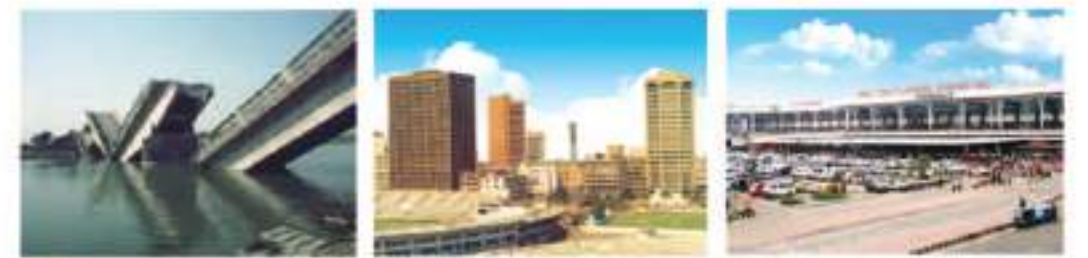
1972 Re-constructed 6 bridges of DHK-CTG Highway damaged in the great liberation war 1980-83 Crafted the skyline of Motiheel C/A by building Shilpa Bank Bhaban, Jibon Birna Tower & Janata Bank HQ 1980 Constructed Main Passenger Terminal of HSA
