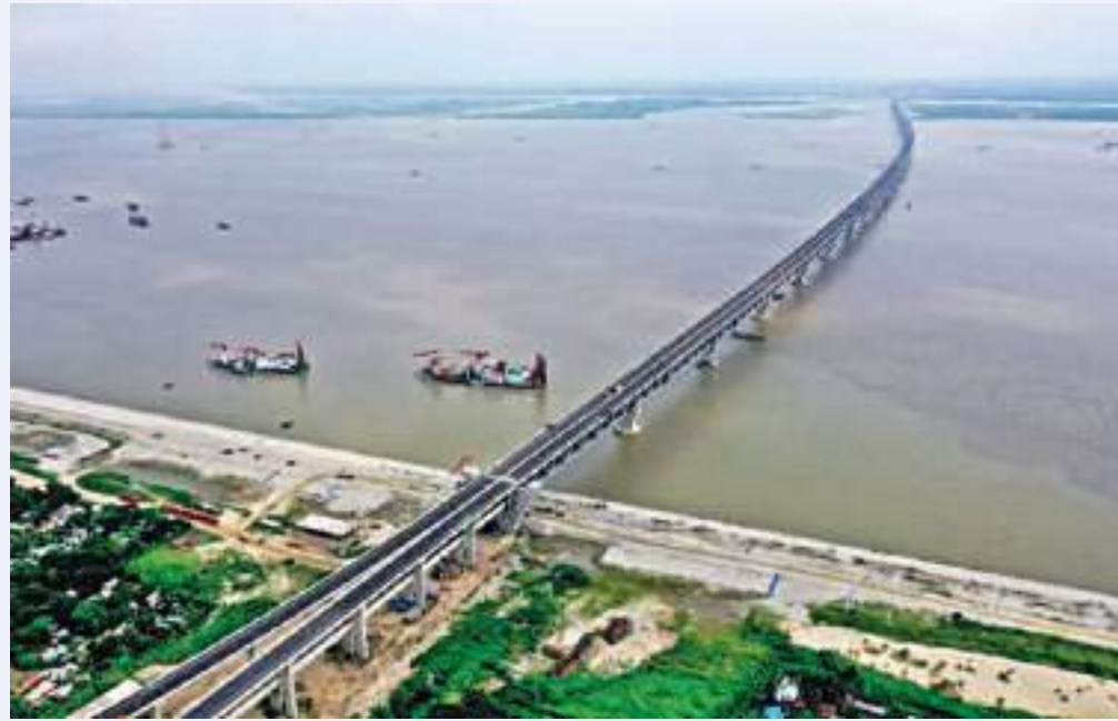
Padma Bridge, the longest bridge in Bangladesh.
